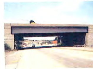
Mainline Bridge (WB-512) over S.R. 0030, Lincoln Highway
