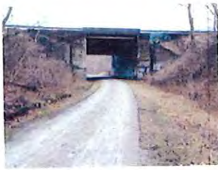
Mainline Bridge (WB-465) over Turtle Creek Industrial Railroad
