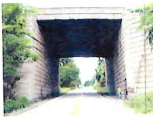
Mainline Bridge (WB-510) over Brush Hill Road
