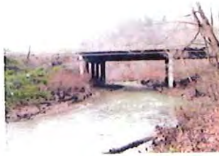
Mainline Bridge (WB-466) over Turtle Creek
