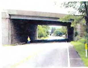
Mainline Bridge (WB-511) over Pennsylvania Avenue
