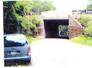
Mainline Bridge (WB-464) over Abers Creek Road
