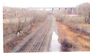
Mainline Bridge (WB-509) over Brush Creek
