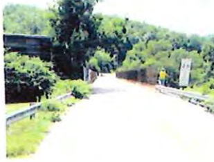
Harvison Road Bridge (WB- 504) over Mainline
