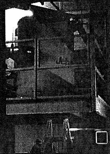
A Jellyfish Filter was constructed from fiberglass to reduce the weight of the system, allowing for a suspended installation above an underground parking structure. The reduced weight eliminated the need for structural changes, and suspending the Jellyfish resulted in no loss of parking space, maximizing real-estate value.
