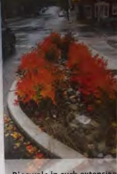
Bioswale in curb extension also provides traffic common and ADA improvements
